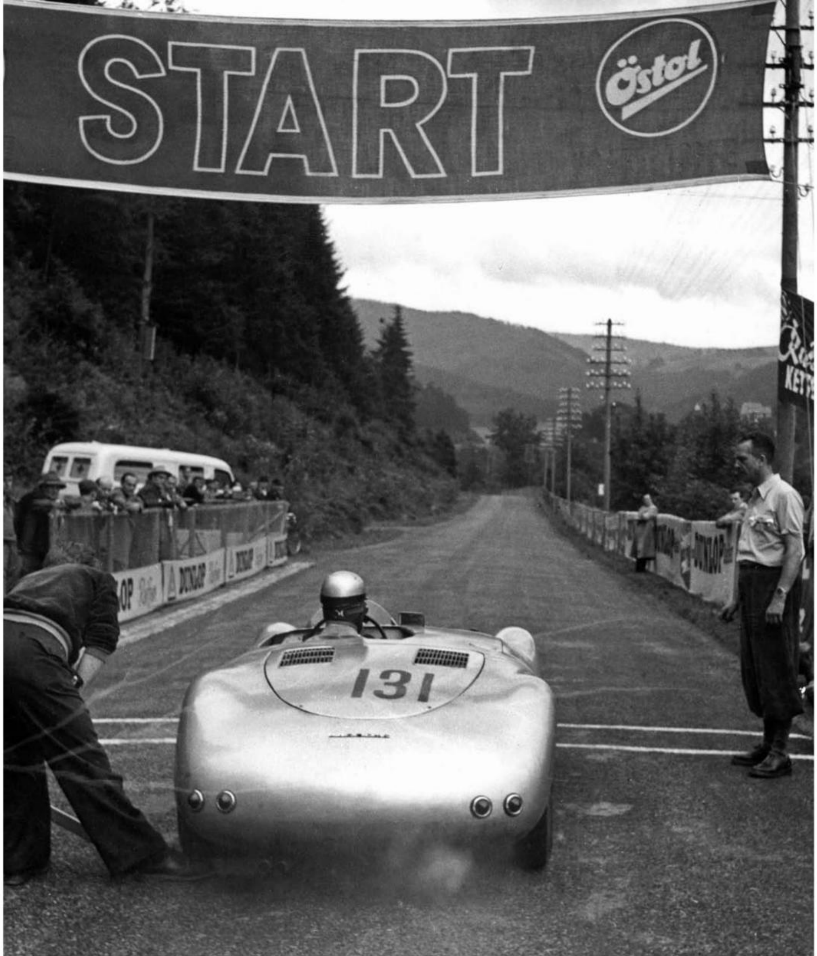
Glöckler and Ramelow created a lightweight 990-pound (450-kilogram) single-seater and used a Porsche 1.5-liter flat-four that they modified to achieve 85 brake horsepower. C. H. Wiedenhausen, a small car-body shop near Glöckler's shops, designed and fabricated the body.
